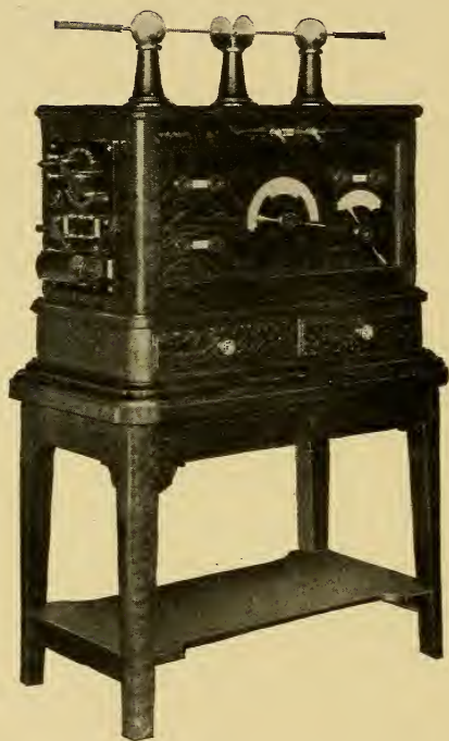
Fig. 1—Large Tesla Coil.
